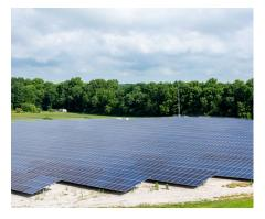
In April 2021, we broke ground on the 40-acre West Plains solar array — the array will be just under 11 megawatts and will be constructed with over 26,000 panels. The site is projected to be completed by Spring of 2022.
