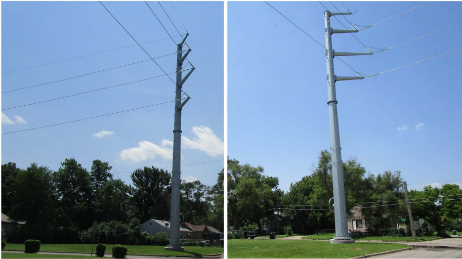
SOUTHEAST CORNER OF MOSSMAN & GREEN - EXISTING
